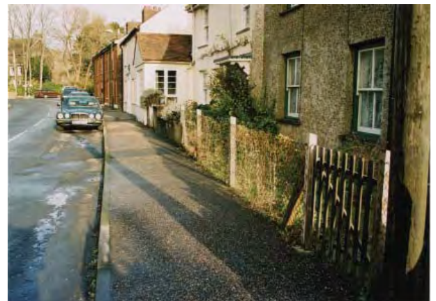
Poor quality front fencing should be discouraged
