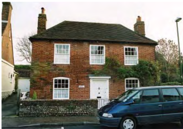
Churchers Farm House, North Street
