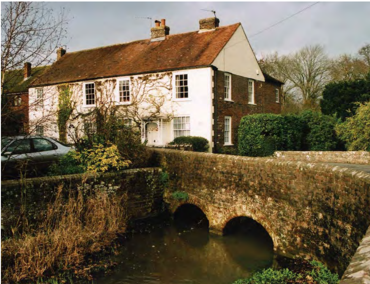
No.56 Commonsides (Bridge House) looks over the River Ems (Area 1)
