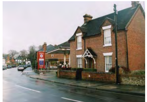
The petrol filling station in East Street is a visually negative site but important for local residents.
