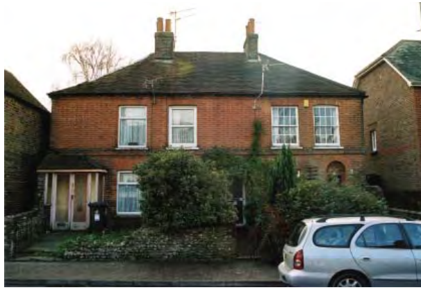
Non designated heritage assets can easily be harmed by the incorrect use of modern materials such as UPVC window frames
