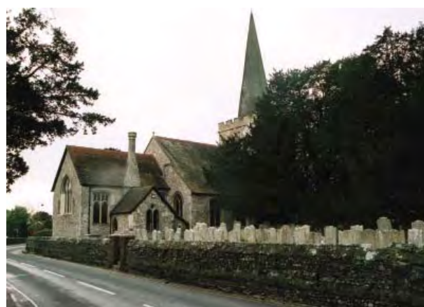
St John the Baptist's Church from Westbourne Road
