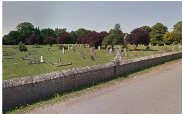
Historic flint and stone walls surround the cemetery, establishing an architectural link to medieval cemetery walls and serving to deter grave robbers.
