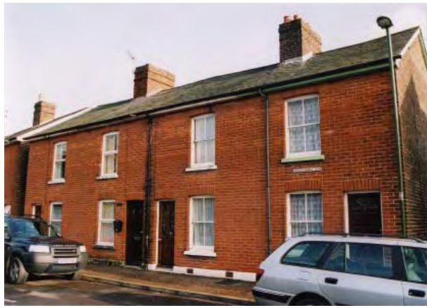
Non designated heritage assets in North Street
